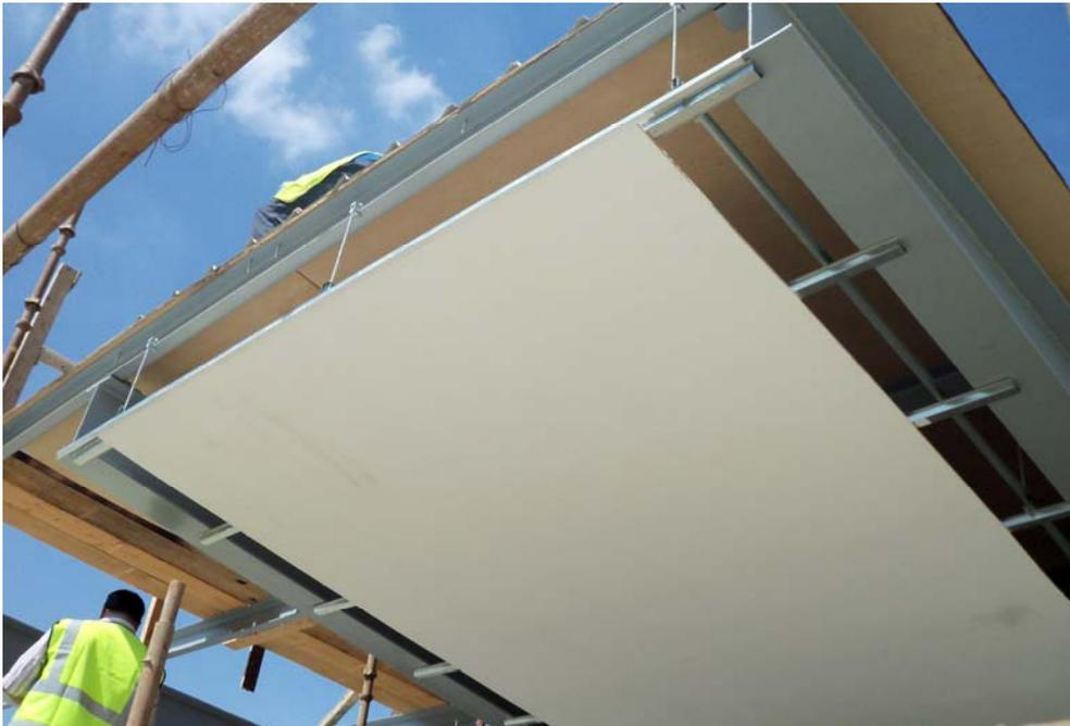
**Fig. 4:** Using Magnesium oxide boards supporting metal frame.
