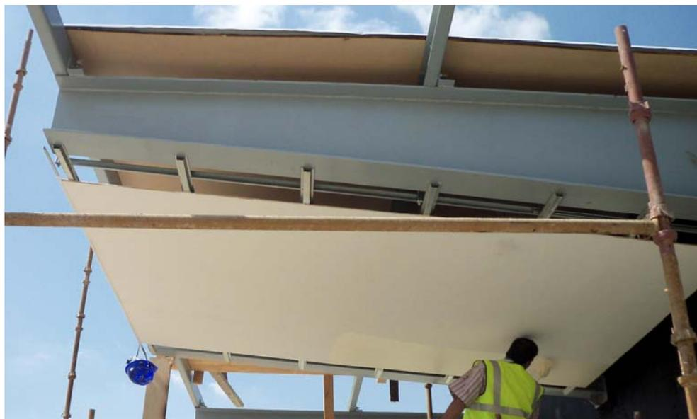
**Fig. 5:** Using Magnesium oxide boards as Ceiling shaping material
