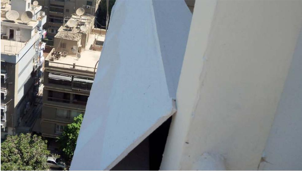
**Fig. 3:** Using Magnesium oxide boards as Building Façade shaping material.
