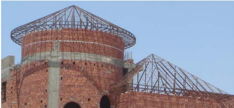
**Fig. 2:** Steel Frame to support Cement plaster on expanded metal lath.
