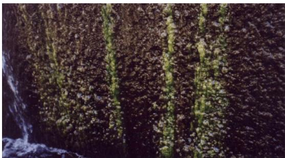
Fig. 1: Algal growth on the wet cemented walls.
