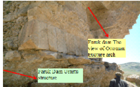
Fig. 9: Faruk dam (2004). Ottoman arch. Urartian construction.
