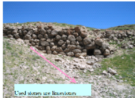
Fig. 5: Dyke of Rusa dam (2004). Used stones are limestones
