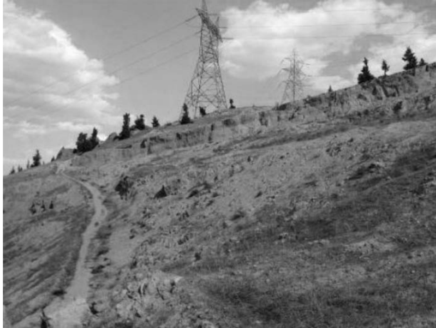
Fig. 1: Landslide near high-voltage power pylons
